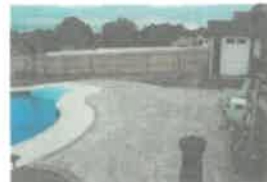
NEW PAVER PATIO 3 PIECE PAVER KIT W/ 6" X 6" BORDER PATIO TO START 3' OFF HOUSE MATERIALS & COLORS INSTALLED MAY DIFFER FROM PHOTO EXISTING FENCE #2 STONE
