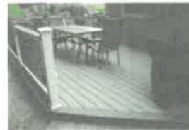
NEW 14' X 20' DECK W/ 10' X 4' LANDING AT HOUSE INSTALL CHICKEN WIRE ON ALL SIDES OF NEW DECK MATERIALS & COLORS INSTALLED MAY DIFFER FROM PHOTO
