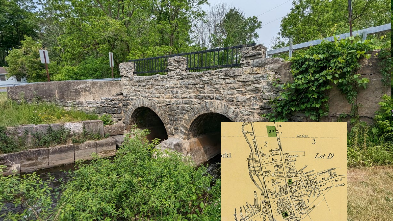
Stone Bridge over Skaneateles Creek in Mottville
