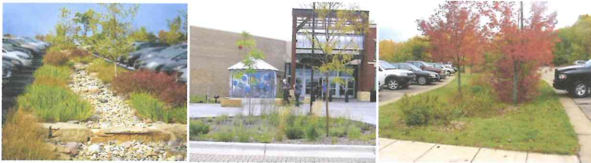
Parking lot infiltration bio-swale at the offices of Novus in St. Louis, with cascades over check dams (left), a landscaped cistern retrofitted at the entrance to Maplewood Mall in St. Paul (center), and red maples planted in bio-swales at H.B. Fuller Company in St. Paul, where the parking lot has no curbs blocking water flow.
