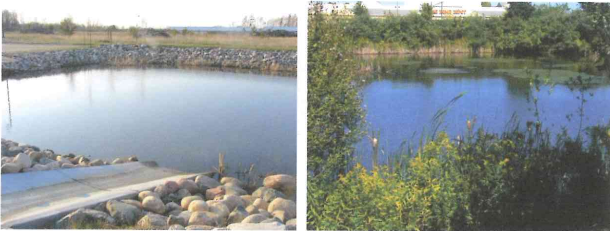
Wet ponds for stormwater retention need not be designed in a sterile way without attractive landscaping, as the above photo pair illustrates. The pond on the right serves a large parking lot and extensive roof area at the Home Depot in North Kingstown, RI. It attracts aquatic wildlife such as ducks and cormorants, in addition to small mammals such as muskrats.
